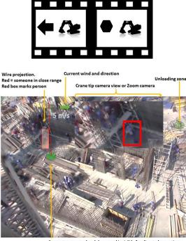
Cargo storage one level down and invisible for direct observation. Green zone marks were and that no person in perimeter
