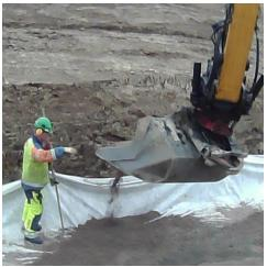
Figure 3 Picture from the cabin of the excavator, showing the ground worker instructing where to pour gravel and how much.
